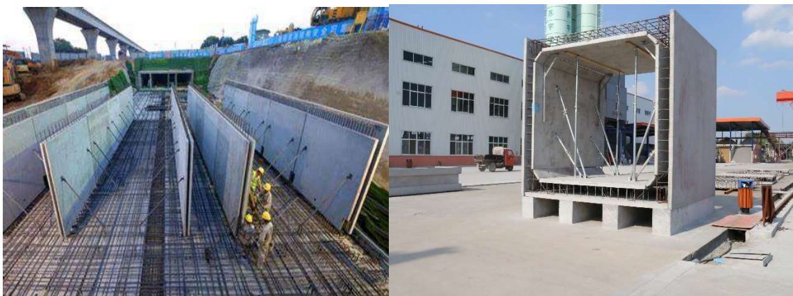
Figure 3. Construction methods of semi-prefabricated utility tunnels
