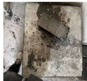
(b) Concrete Vibration
