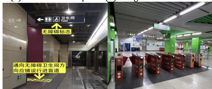
(c) Break in tactile paving
